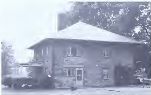
Home near U.S. Route 322, east of Hummelstown; once a carriage house; limestone and brown sandstone.
